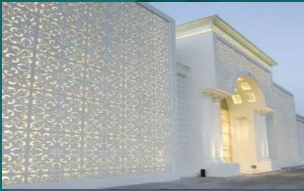
EXTERIOR WALL DECORS
